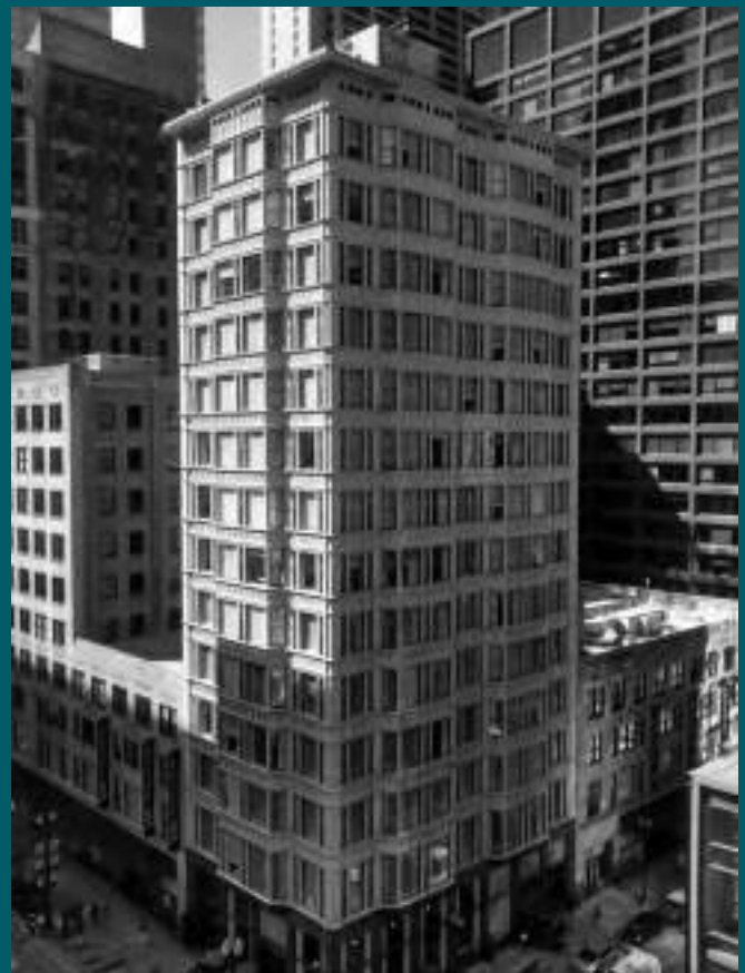
Reliance Building, 1895, Daniel Burnham, Chicago, Illinois © Mx. Granger
